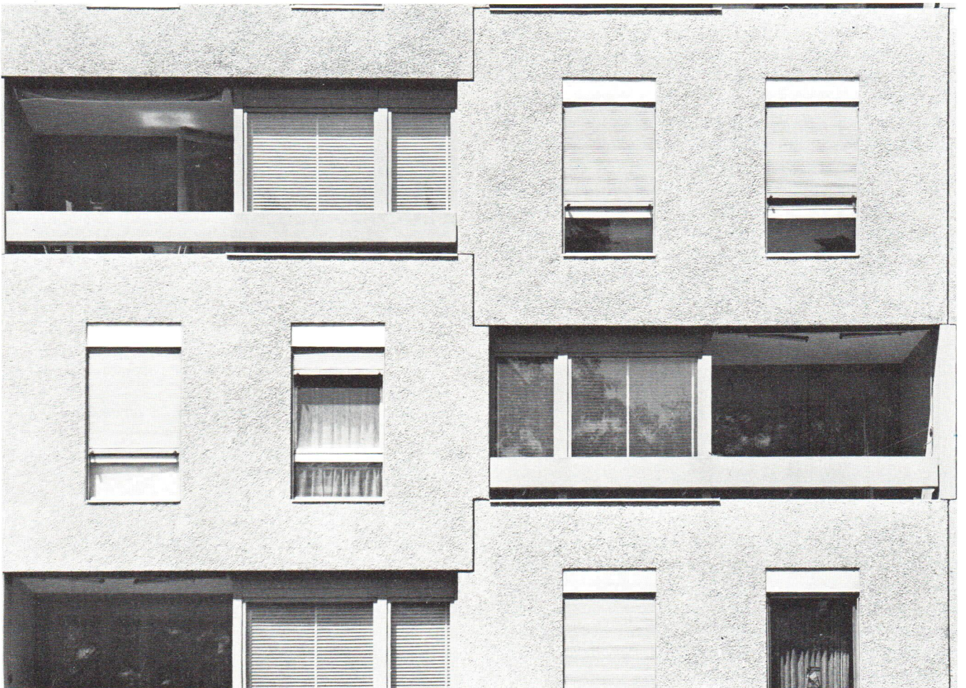
Various developments of window parts Igeco system. Contrasting play of different types of surface structures (smooth moulded concrete, washed concrete, etc.) and proportions
