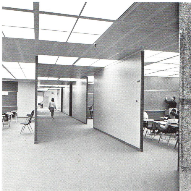
Flexible plans by means of movable partitions. SCSD (School Construction System Development) of the State of California Flexible Grundrisse durch verschiebbare Wände. SCSD (School Construction System Development) des Staates Kalifornien, USA Plan flexible, cloisons mobiles. SCSD (School Construction System Development) de l'Etat de Californie, USA
